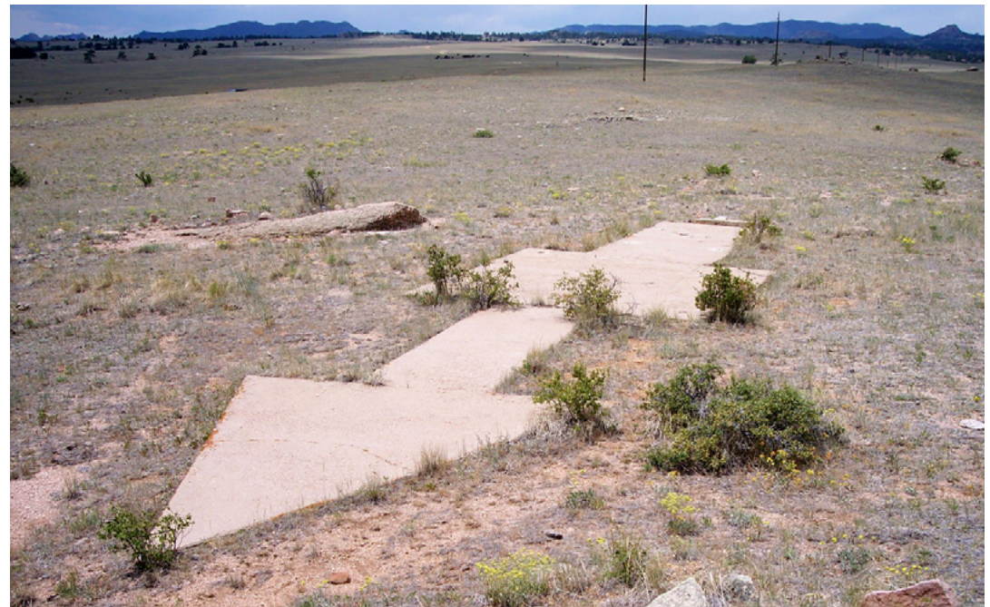
Standard airway beacon installation of 1931 from ATCHistory.com
